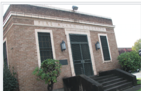
Fire Alarm Telegraph building in the Kerns neighborhood of Portland
